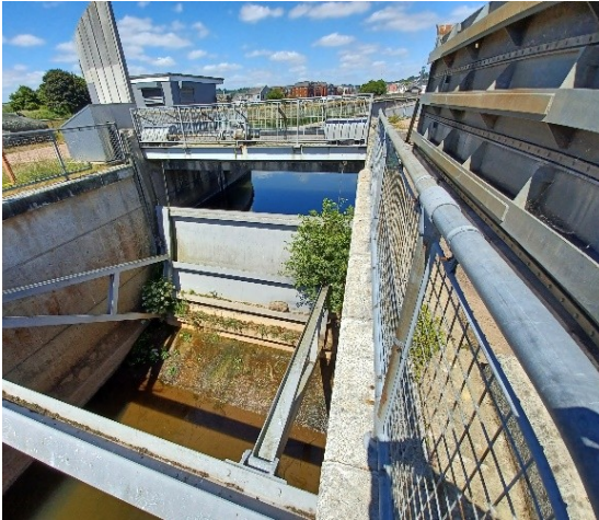
Figure 2 - The radial gate at Trew's Weir.
